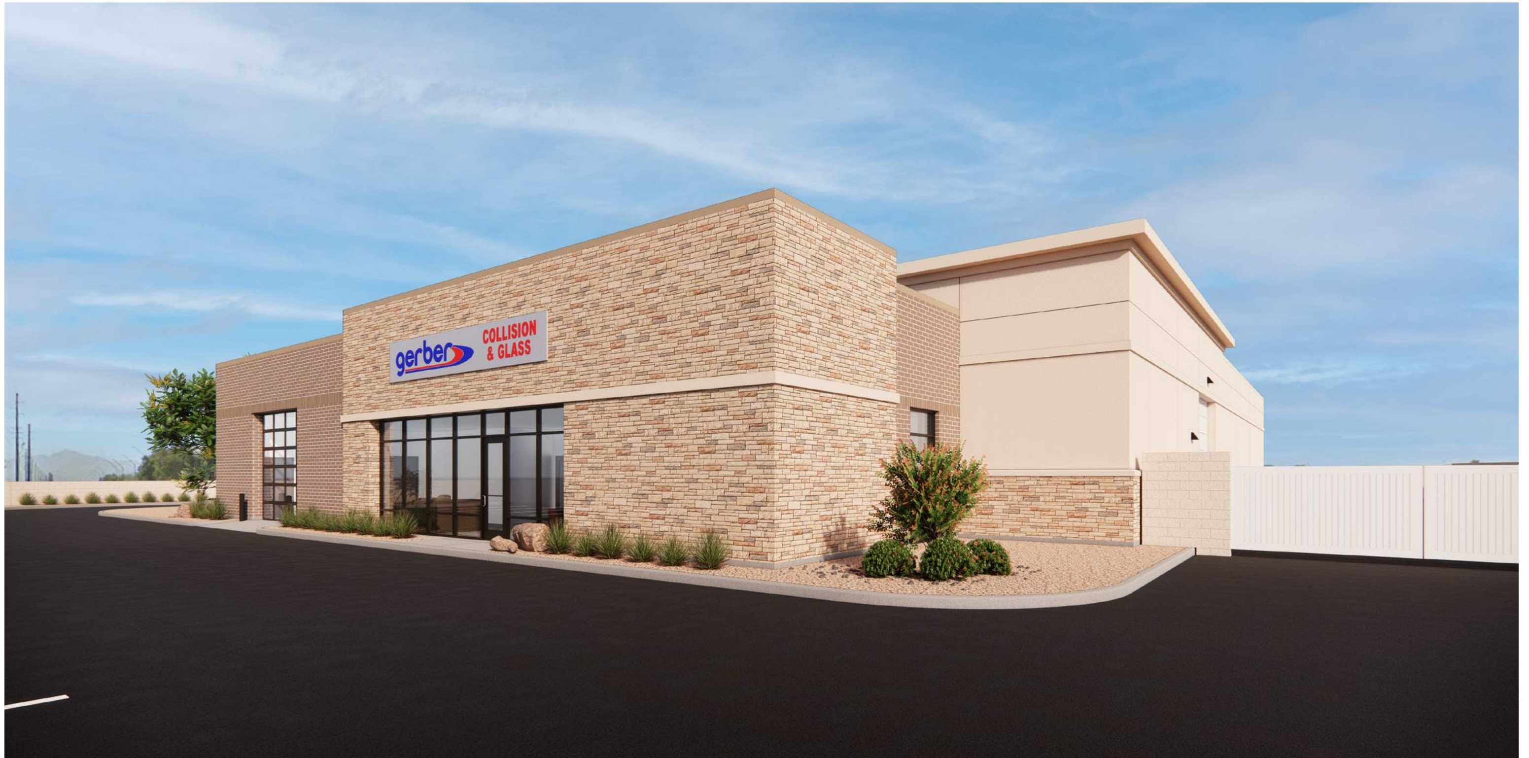
Corner of North/East Elevations & Fence
